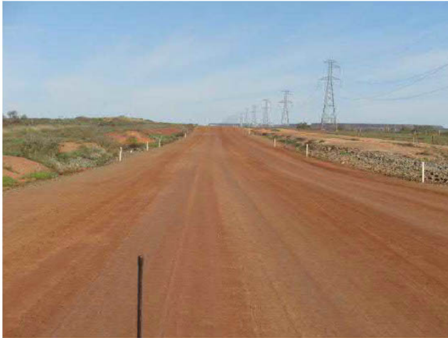
Picture 1 - Typical Haul Road / Floodway
